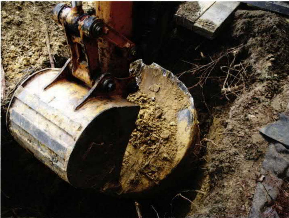
Picture 2: UST 1293Eagle removal in progress.
